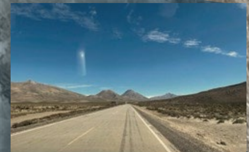
Paved Highway to site
